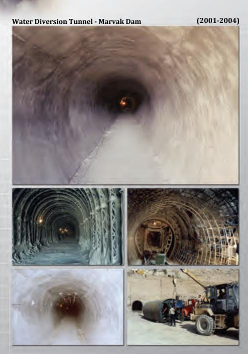
Including implemeting and excavation and lining of the two Tunnel, each 500 meter long and two vertical and one angled shaft (total length:120 meter) and their subordinate structures in beginning along and at the end of the part and also Pre-Constructing the camp and landscaping of the camp.
